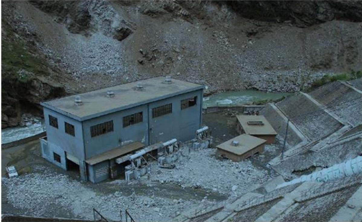
*Upper Bhotekoshi hydro power plant damaged by earthquake-induced landslide. (Photo courtesy: IPPAN)*
