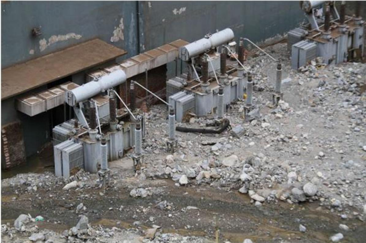
*Upper Bhotekoshi hydro power plant damaged by earthquake-induced landslide. (Photo courtesy: IPPAN)*
