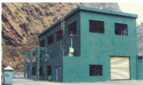
Upper Bhote Koshi Hydroelectric Plant - Powerhouse
